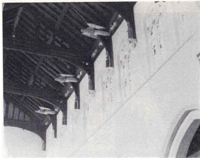
View of Nave Roof
